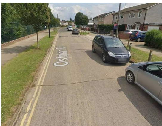
Figure 6. Concrete Slab Surfacing
